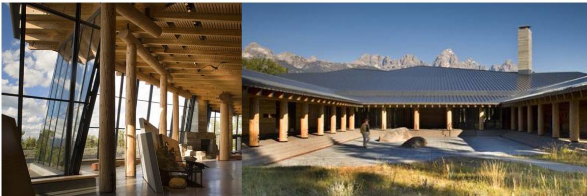
Figure 33: Examples of glulam timber at the Grand Teton Craig Thomas Discovery and Visitor Center. Image source: Nic Lehoux.
