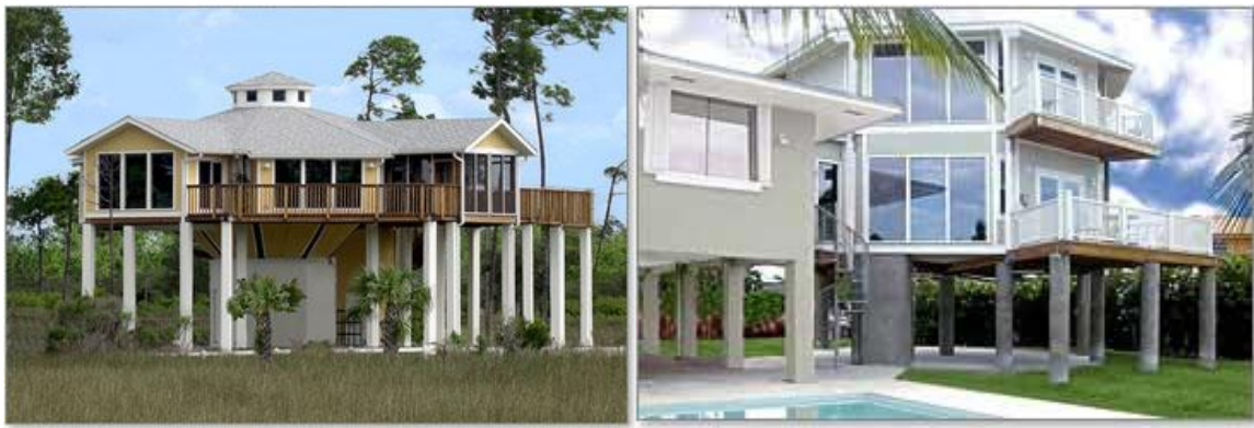
Figure 32: Examples of concrete piles in Gulf Coast houses. Image source: Topsider Homes.
