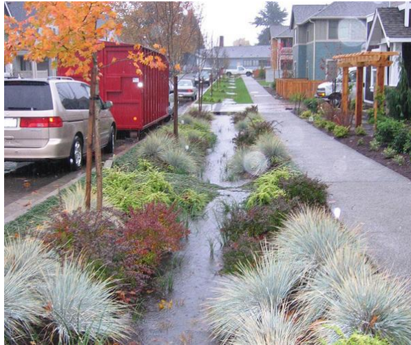
Figure 14: A bioswale - a common example of green-blue infrastructure in urban environments.
