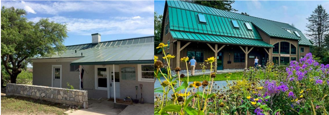
Figure 36: Examples of nature centers with standing seam metal roofs. Image sources: Eaton Hill Nature Center and Hauser Nature Center.
