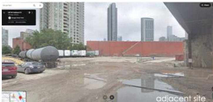
Figure 8: West side wall (visual: Google Maps)
